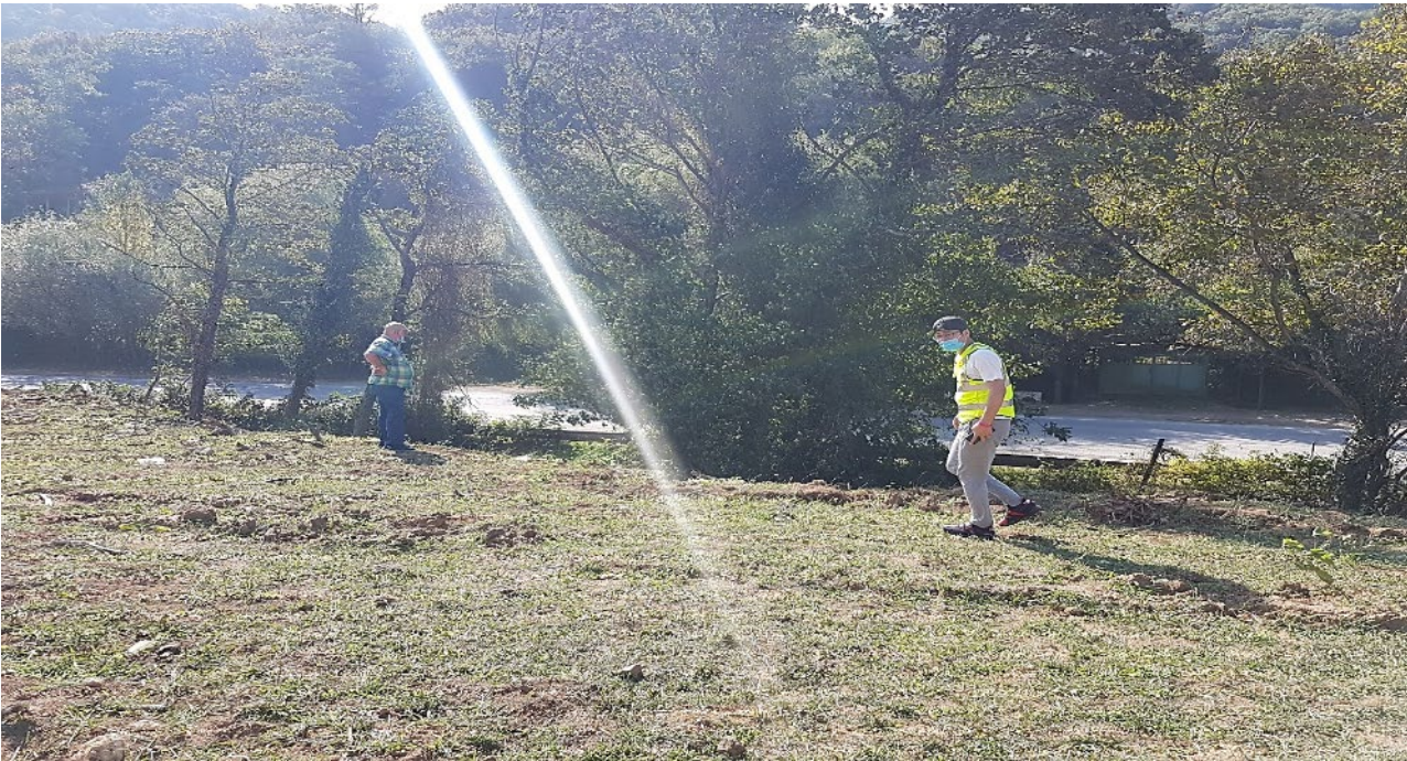
Visit the site to explore the issue of damage to the fence of local resident’s private land fence
