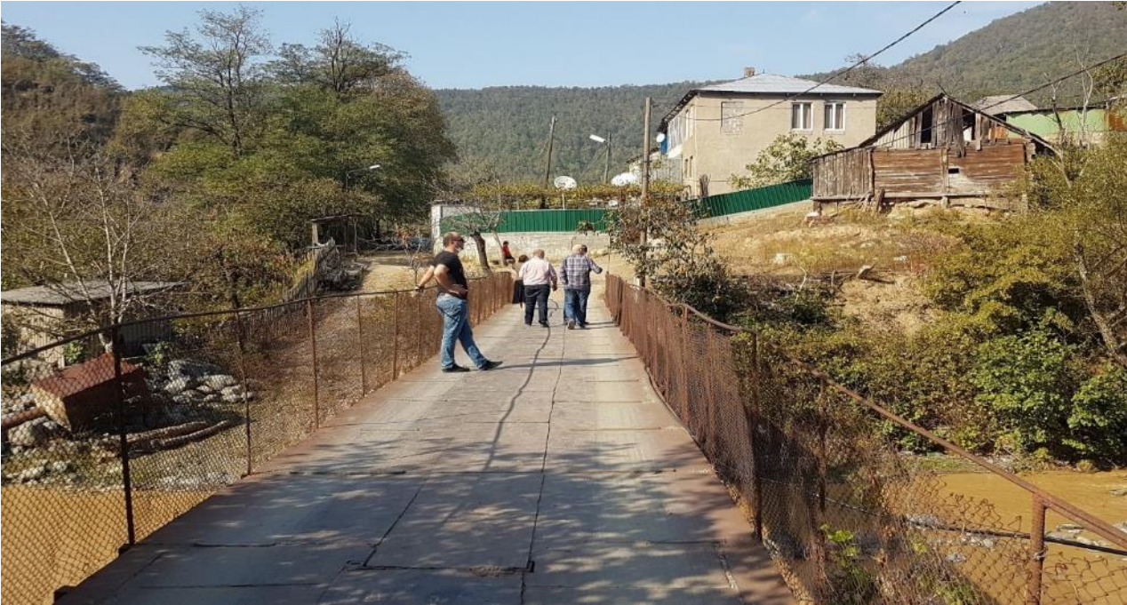
Visit the site to explore the issue of blocking one of the access roads to the local settlement in the process of arranging the western portal of tunnel N6
